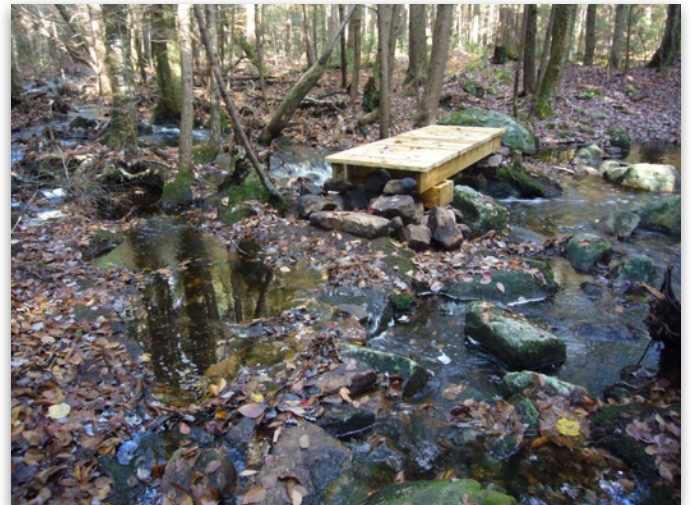
New bridge on Morgan Hill Trail
